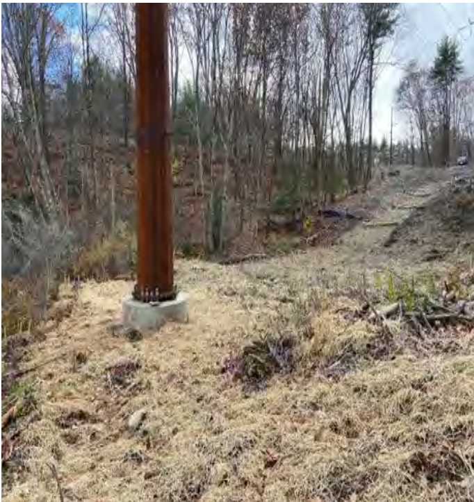
Fig 3: Str. 28 restored work pad. Viewing southeast. (11-08-19).
