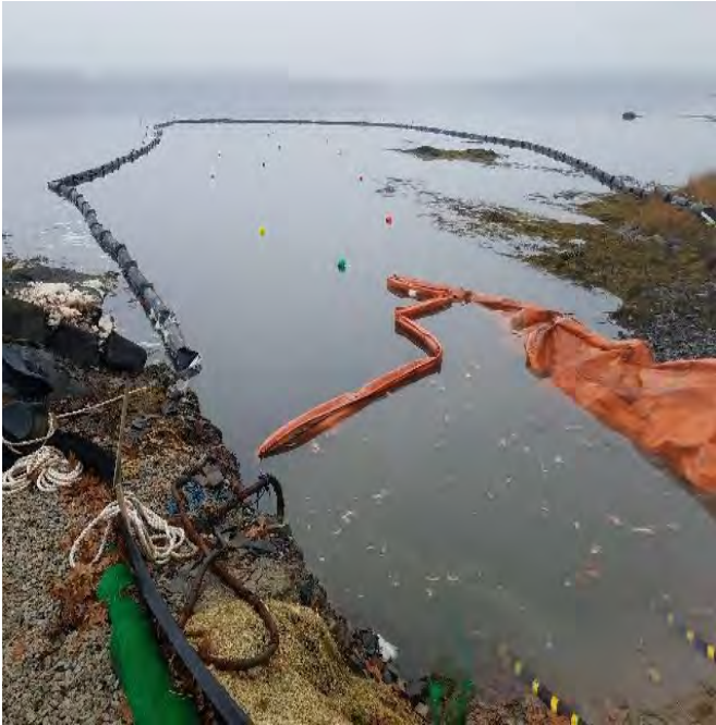
Fig 5: Turbidity curtains installed at the Getchell property/west side of the bay. (11-12-19).
