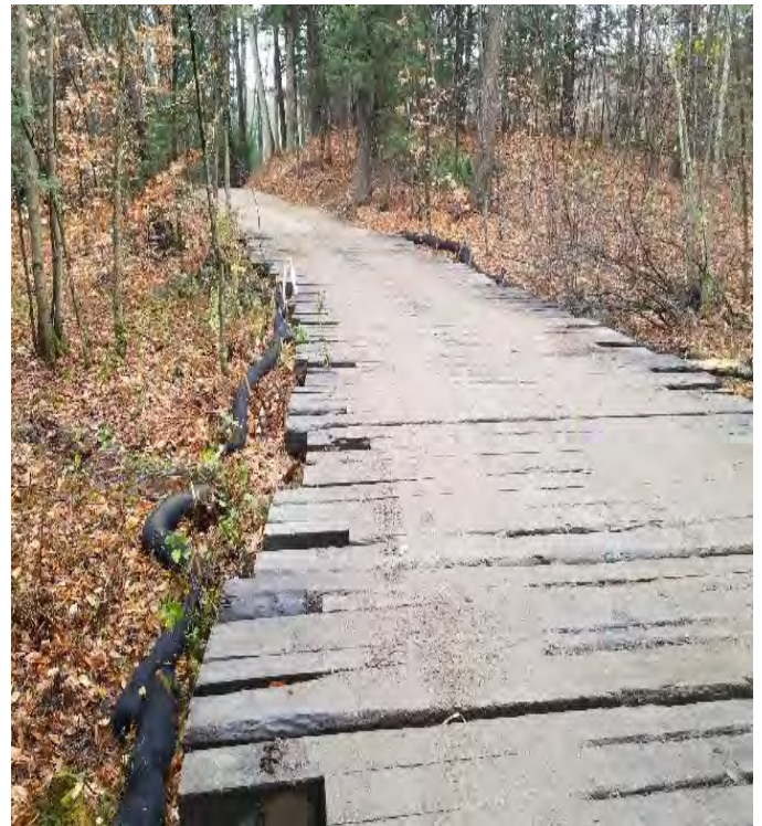
Fig 10: Filter sock installed on access road off of Route 4. Viewing east. DW 202. (11-12-19).
