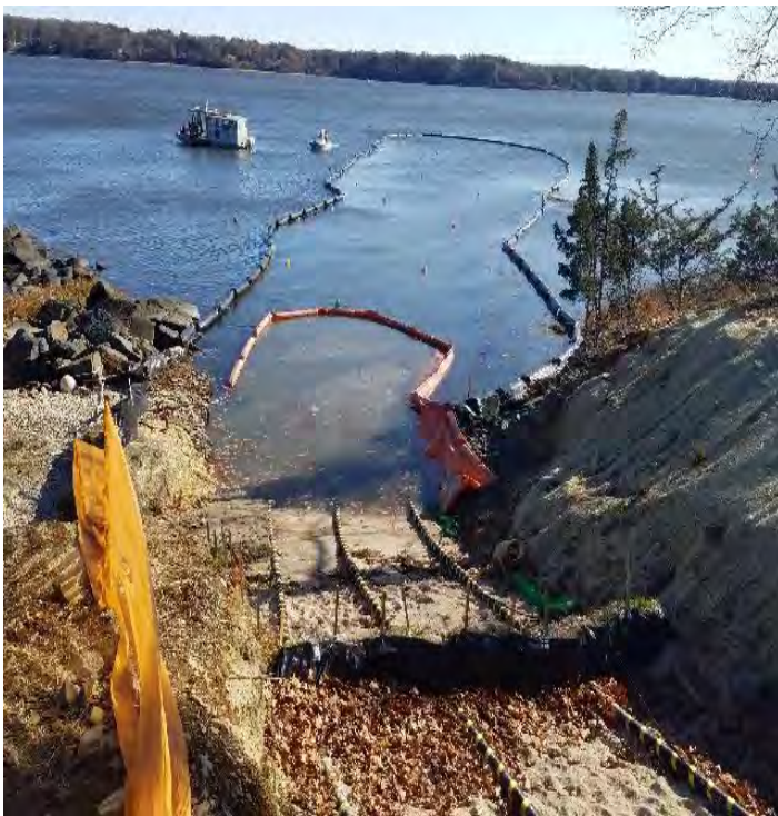
Fig 11: Turbidity curtains installed at Getchell property/west side of the Bay. Viewing east. (11-13-19).
