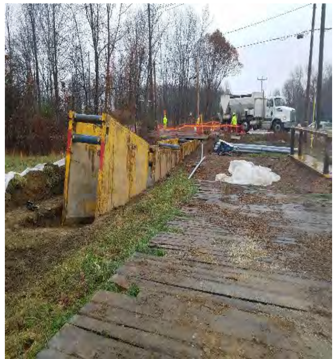
Fig 8: Trenching under Nimble Hill Road. Viewing west. (11-12-19).
